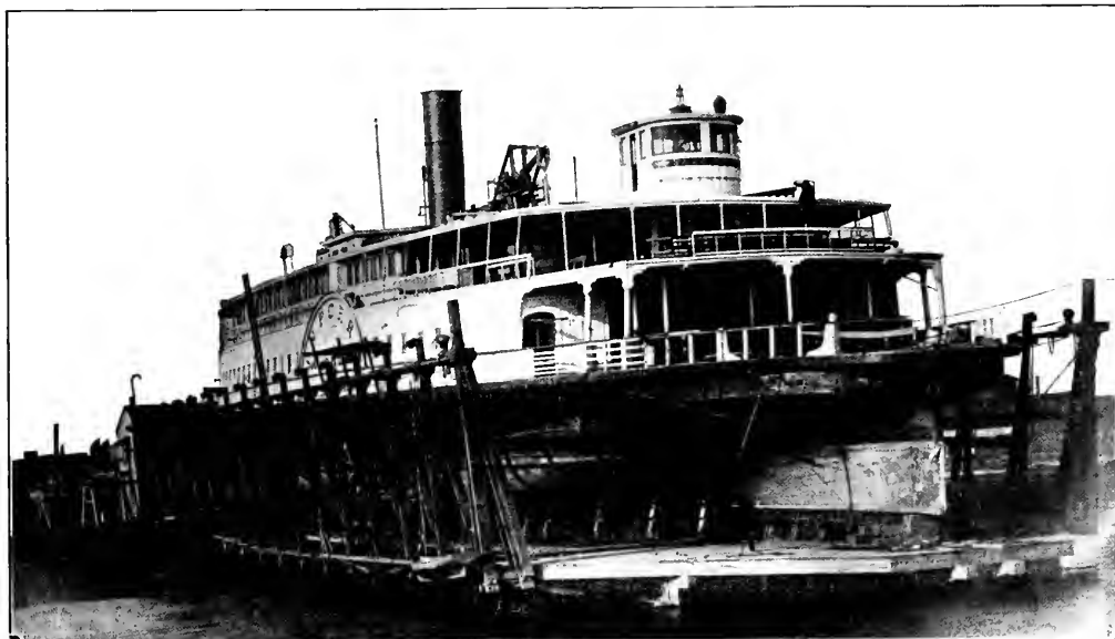
A 2500-ton Crandall dry dock with the ferryboat "Sausalito." These docks are well represented all along the West Coast.
